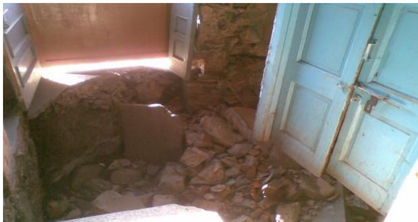
Fig. 1: Sinking of floor
