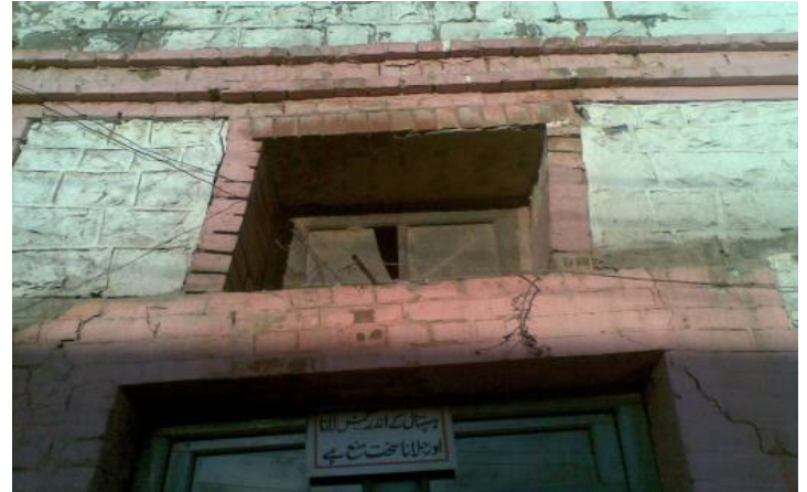
Fig. 4: Sway of front wall
