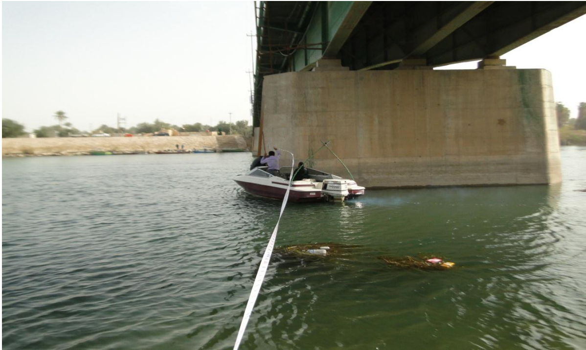
Figure (3): Measuring the geometric bridge data
